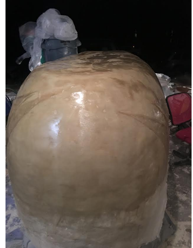
Fiberglass laid over mold
